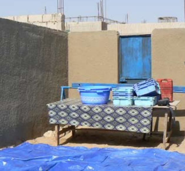
The Cooperative rented a new production workshop that is more spacious, wired for electricity and easily connected to running water. The workshop is made up of three painted rooms with cement floors and a sandy courtyard.
